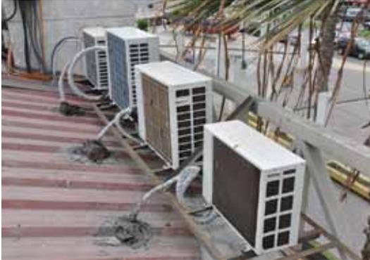
**Figura 4103.** Conexión a la estructura de soporte de aire acondicionado
